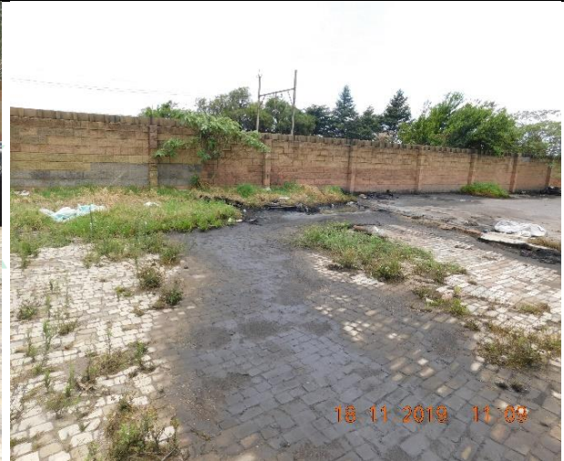
Figure 10: Oil spillage onsite.
